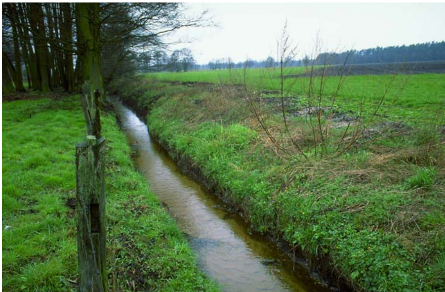
Fig. 4: The Endeholz Ditch in spring of 1998 after management by machines. On the right side the excavated material can be seen. The river bottom is exclusively sand. The ripples are characteristic of the moving sand.
